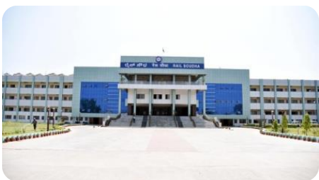
❑ South - western railways headquarters
