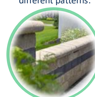
Stone cladding on toe walls along walkway and cycle tracks for seating
