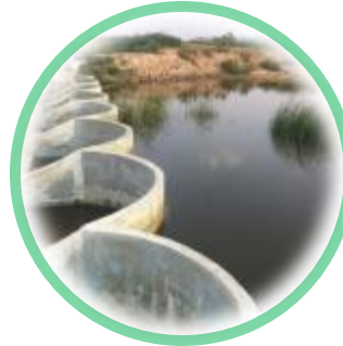
Multi arched check dams with walkway
