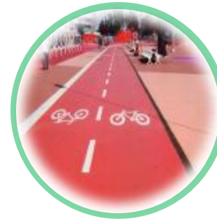
PCC pavement with paint finish
